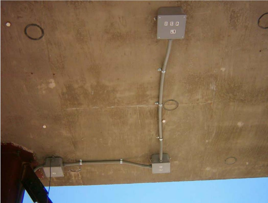
Figure8. Top slab sensor enclosures
