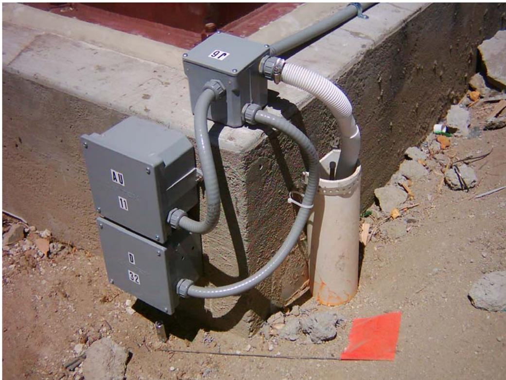
Figure7. Bottom slab corner with vertical accelerometer, displacement, and soil pressure instrumentation
