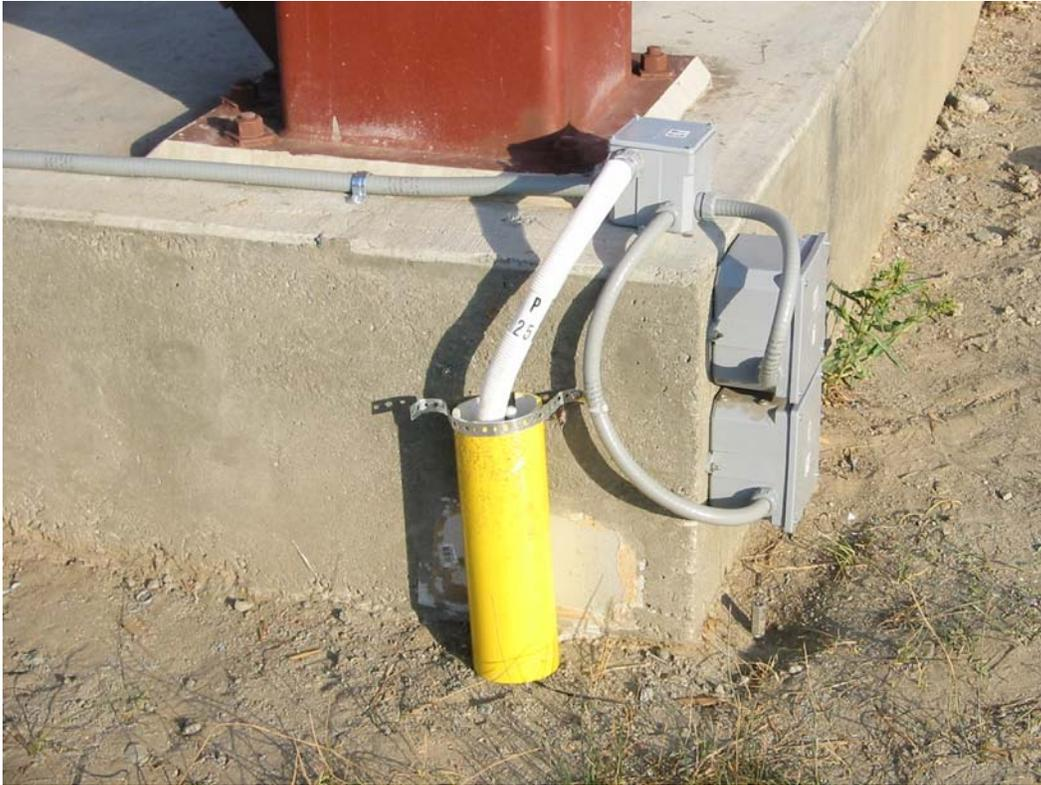
Figure6. Bottom slab NW corner, showing displacement sensor
