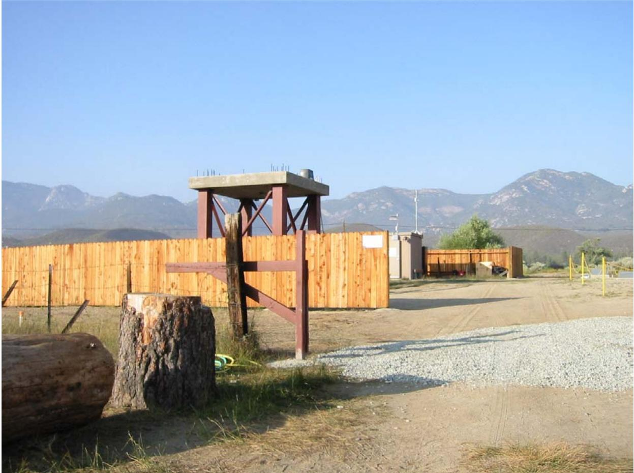
Figure3. GVDA entrance, showing gate, fence, SFSI structure, and instrumentation building
