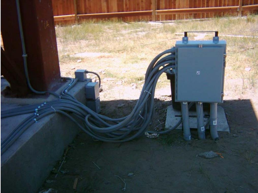
Figure9. Main cable junction box
