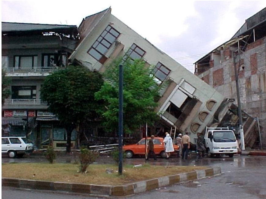
Figure 2-2 Liquefaction-induced bearing capacity failure of a 5-story building in Adapazari following the 1999 Kocaeli, Turkey earthquake (from [www.eerc.berkeley.edu/turkey/adapazari](http://www.eerc.berkeley.edu/turkey/adapazari)).
