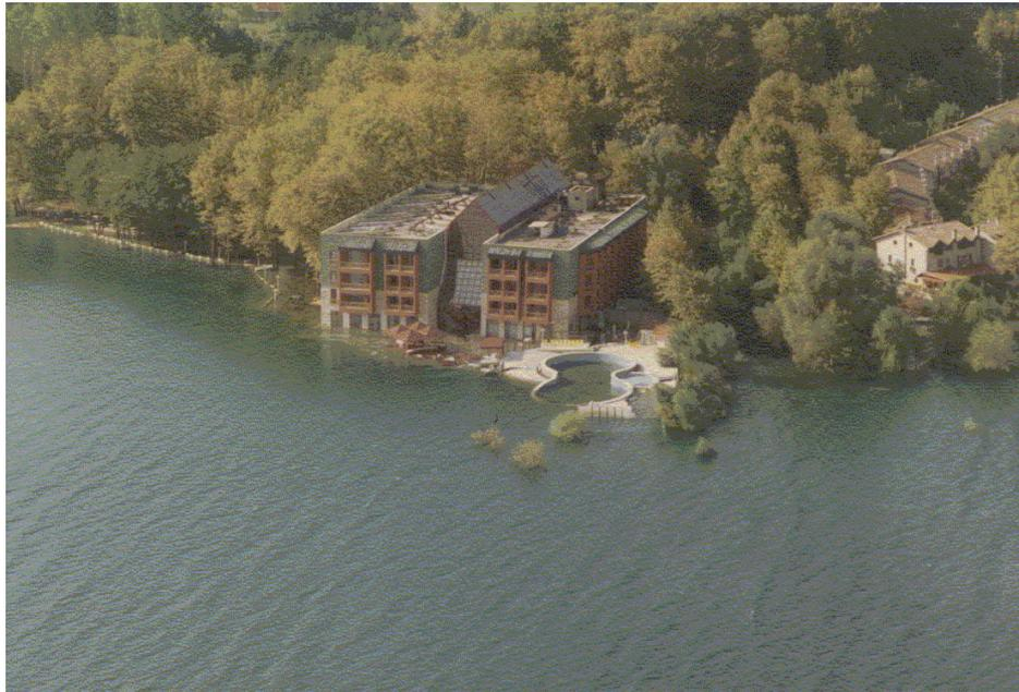
Figure 2-3 Liquefaction-induced lateral spreading and settlement, coupled with tectonic subsidence, carried Hotel Sapanca partially into Lake Sapanca following the 1999 Kocaeli, Turkey earthquake (from [www.eerc.berkeley.edu/turkey/adapazari](http://www.eerc.berkeley.edu/turkey/adapazari)).
