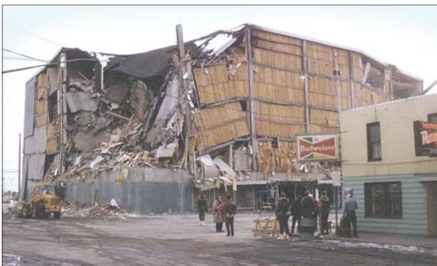
*Wreckage of the J.C. Penney department store, Fifth Avenue and D Street, Anchorage. Building failed after sustained seismic shaking during the 1964 earthquake. At the time this photograph was taken, most of the rubble had been cleared from the street. USGS photograph by George Plafker.*
