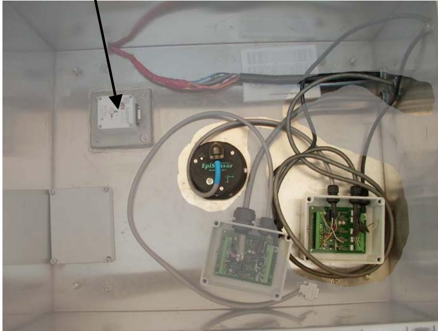
NOTE: The cabling from the sensor to the LP board in the wellhead box uses color-codes from the legacy GVDA wiring where “black” was the positive!
